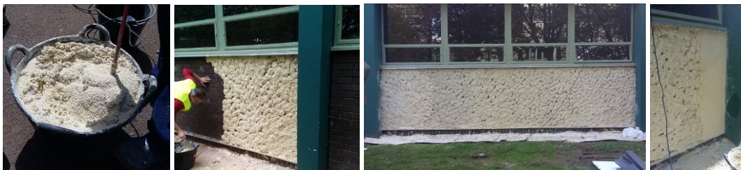
Figure 12: Installation of the aerogel mortar
