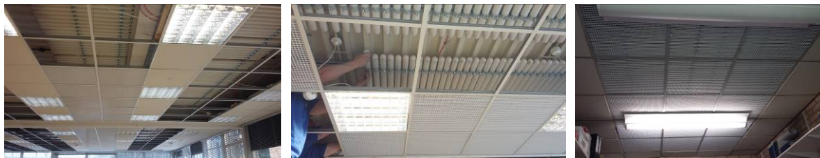
Figure 8: Installation of the PCM tubes
