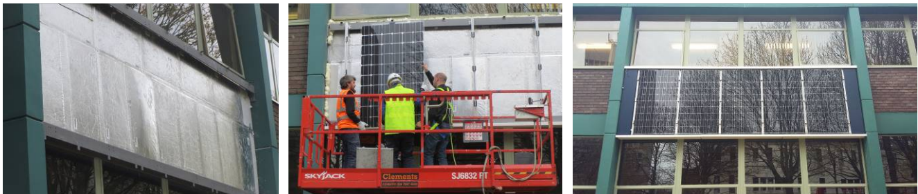
Figure 11. Installation of the ventilated façade
